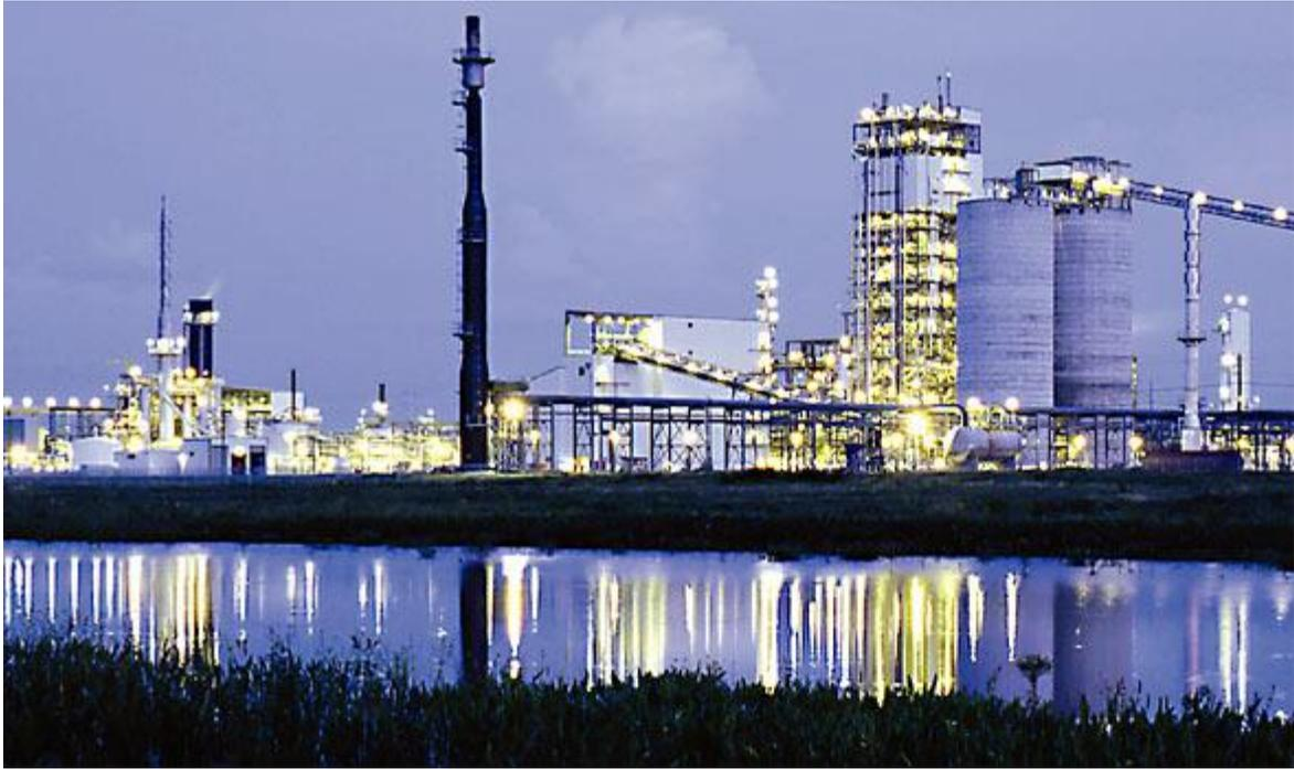
**Figure 7** This power plant in Florida is leading the way in cleancoal technology. The plant turns coal into a gas before it is burned, so fewer pollutants are released.
